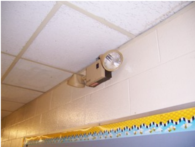
Hallway Egress Lighting
