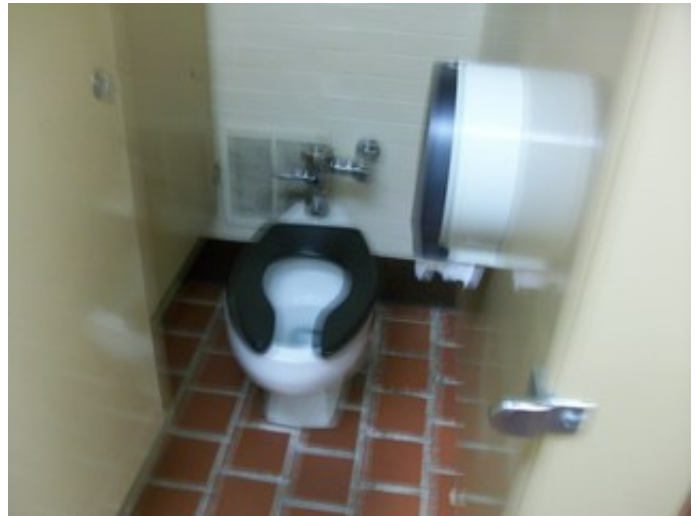
Toilet room fixtures
