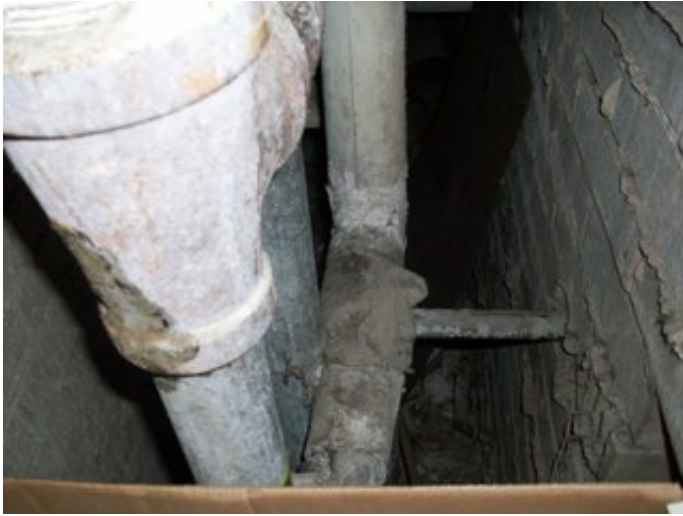
Sanitary drainage Piping
