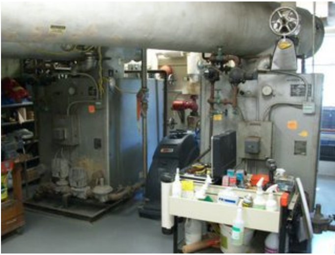
Gas Fired Hot Water Boilers
