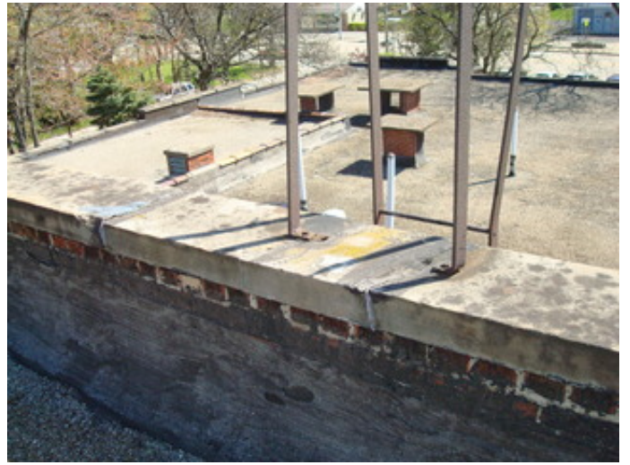
Typical flashing, coping, and roof ladder.
