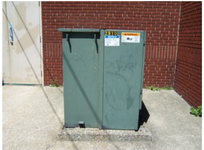
Main Electrical Transformer
