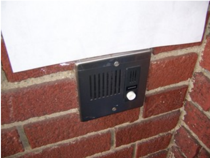
Front Door Wall Mounted Intercom
