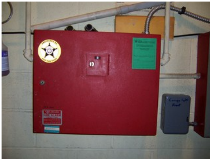
Main Fire Alarm Panel
