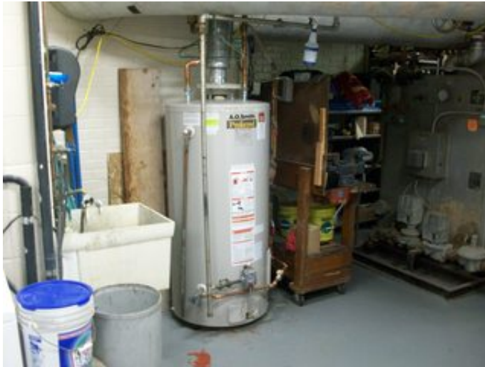
Domestic water heater
