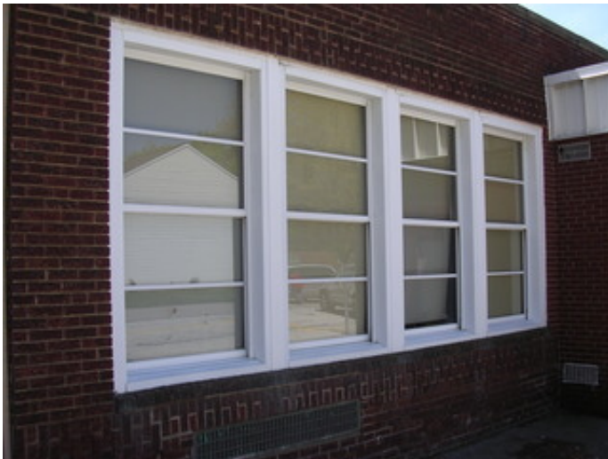
Typical replacement single glazed aluminum windows.
