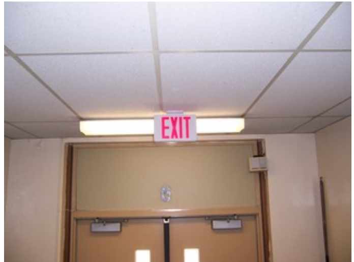
Typical Exit Sign
