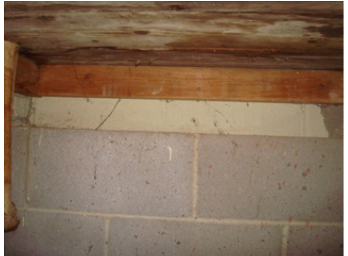
Crawl space wall
