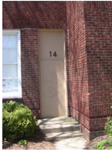
Typical classroom egress door.
