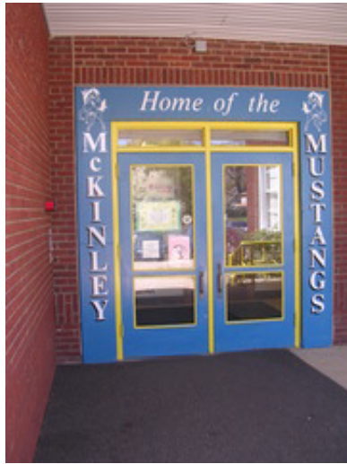
Typical hollow metal entry doors.
