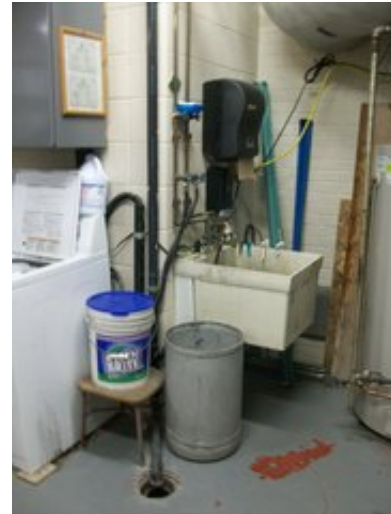
Domestic water piping
