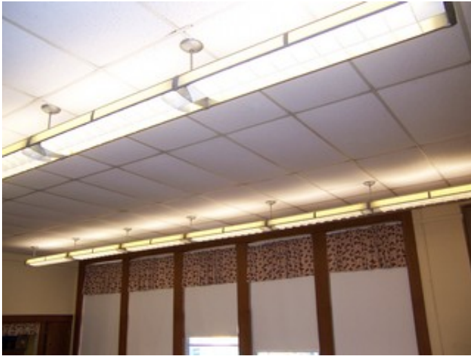
Classroom Lighting Fixtures
