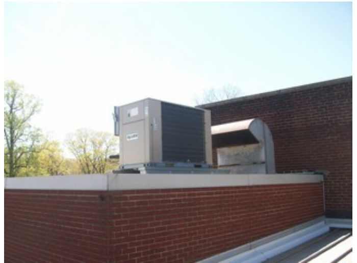
Rooftop Remote Air Conditioner Unit
