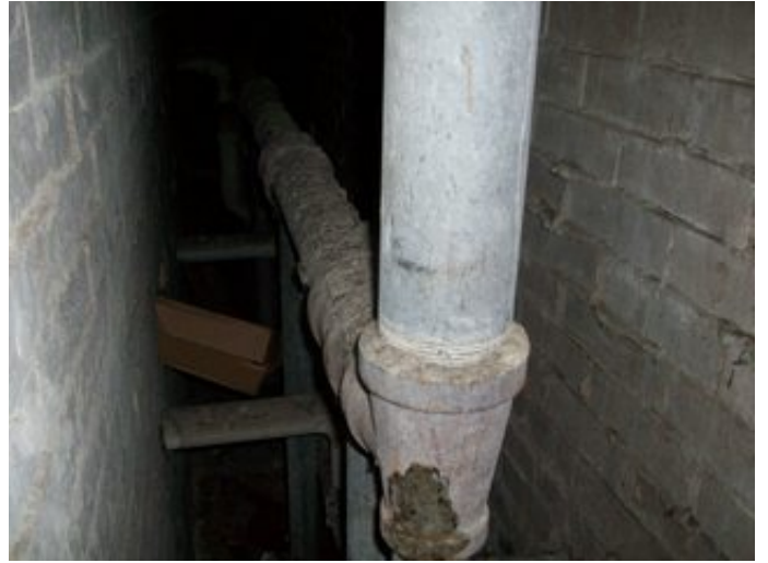
Sanitary drainage Piping
