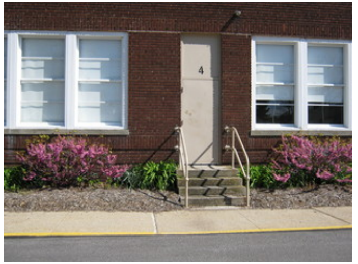
Exit steps at classroom
