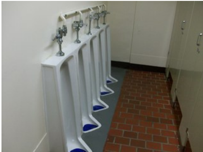
Toilet room fixtures
