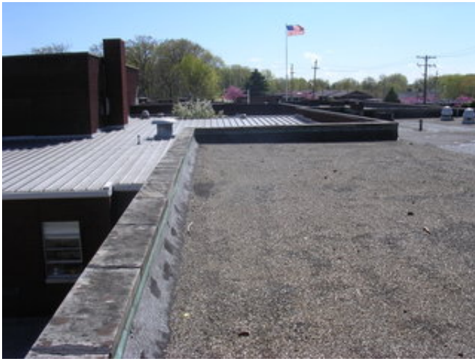
Typical roofing conditions,
