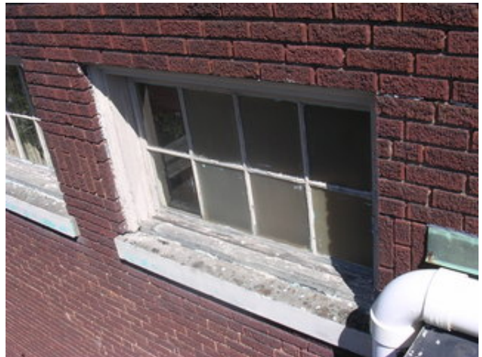
Typical wood windows.
