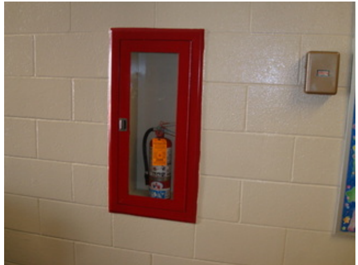
Fire extinguisher cabinet
