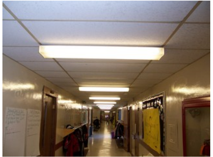
Surface Mounted Hallway Lights
