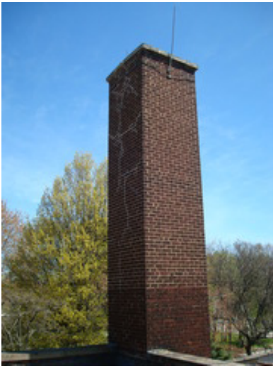
Chimney showing extensive deterioration
