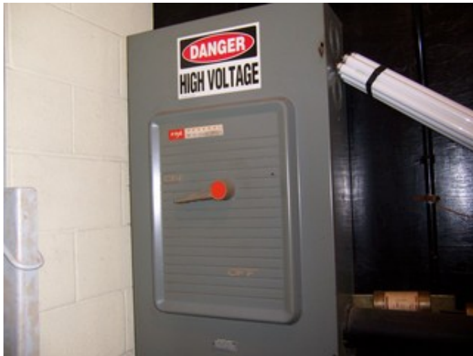
Main Electrical Utility Switch
