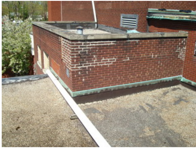
Deteriorated brick near courtyard
