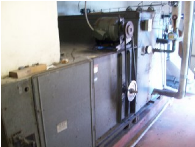
Air Handler Unit
